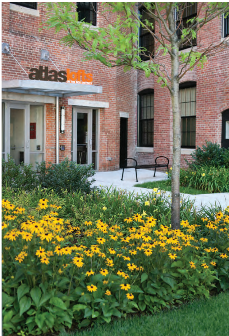
The building that used to house the bedding factory has been transformed into Atlas Lofts condominiums.
